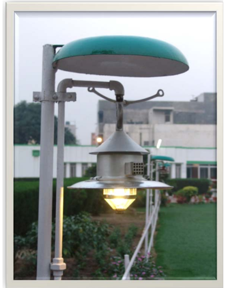
Biogas used for lighting of mantle lamps
