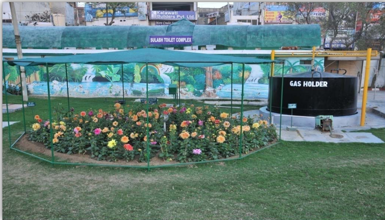
Public toilet linked to biogas plant with gas holder
