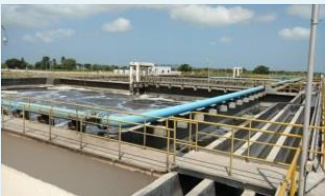
70 MLD STP based on ICEAS Technology for JMC at Jamnagar
