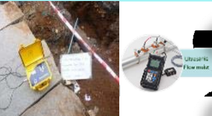
(6) Installation of temporary Flow meter
